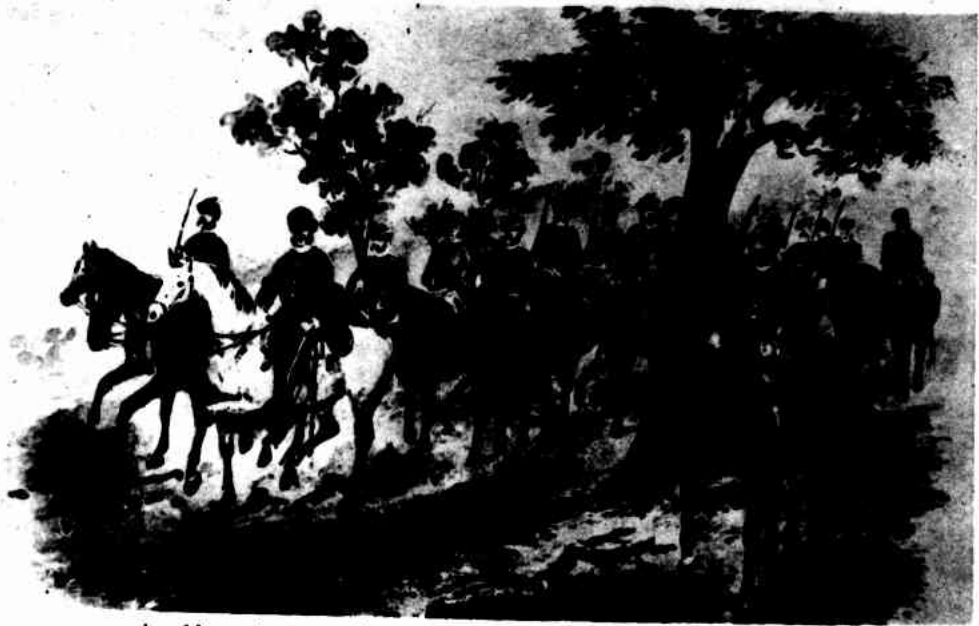
A gold escort sets out from Castlemaine on the road to Melbourne.
